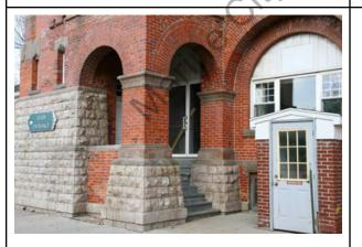
Fig 4. Detail of south west porch, window treatment and contemporary basement access door.
